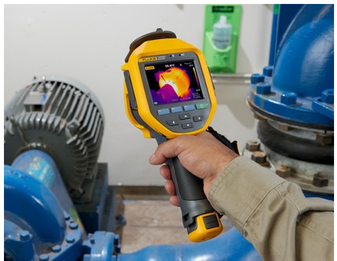
Take a baseline image of all motors, to compare over time, and then routinely look for abnormal hot spots on the motor, under full load.
